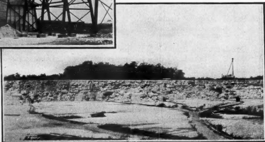
Above is shown the crusher plant at the Rockwell Lime Co., Francis Creek, Wisconsin. The photograph at the right shows the south side of this unusually interesting quarry which employs a Cyclone in drilling operations. The present quarry occupies an area of about 6 acres with a face of about 28 feet.
